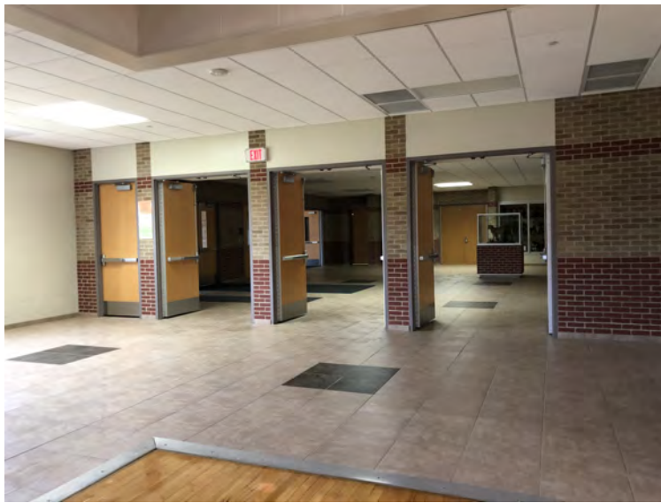
Exit from performance gym back to prop storage area. Same doors as entrance. Each door is 8 ft x 6 ft.
