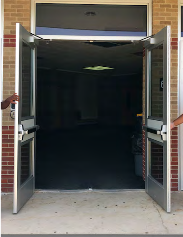
Prop entrance into building 8 ft x 6 ft with center bar removed
