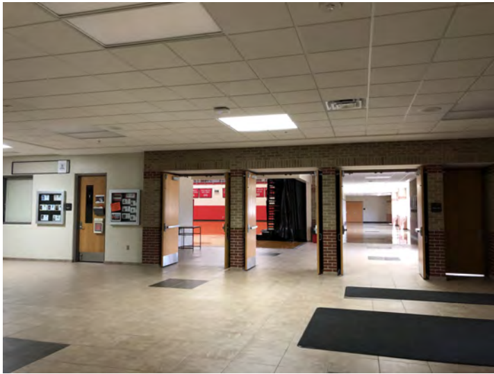
Doors leading into the performance gym entrance at the end of the hall from prop storage area. Each opening is 8 ft x 6 ft with no center bar.
