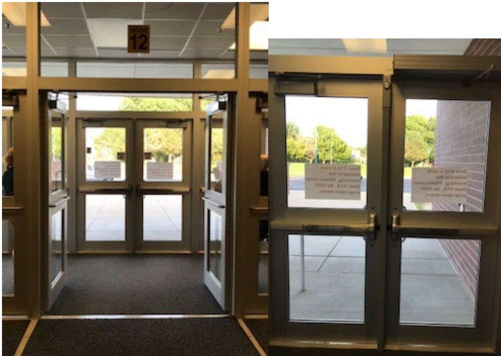
Exit Doors – center bar will be removed Height - 84" Width - 64"
