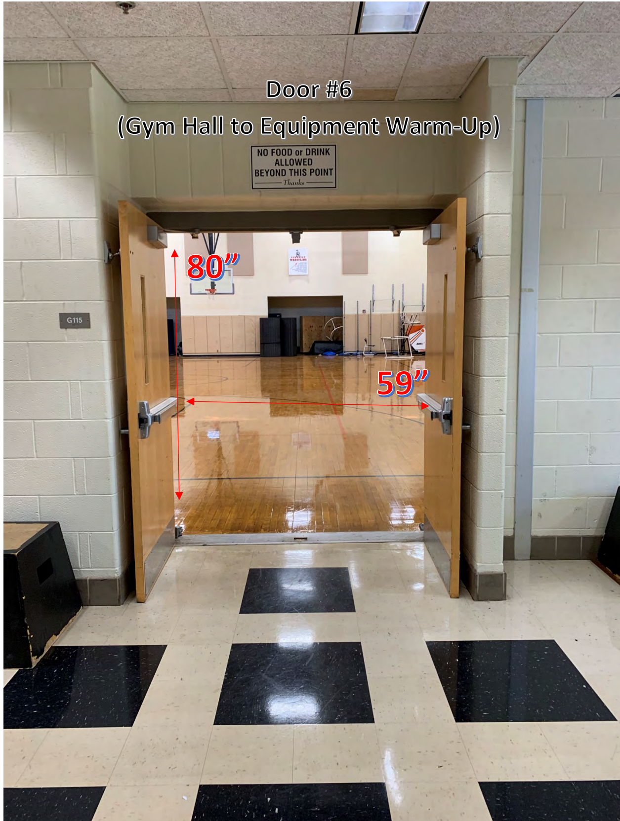
Door #6 (Gym Hall to Equipment Warm-Up [Aux. Gym])
